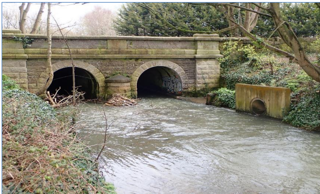
Plate 5: Balheary Bridge (RPS 340; NIAH 11335018) from the East.
