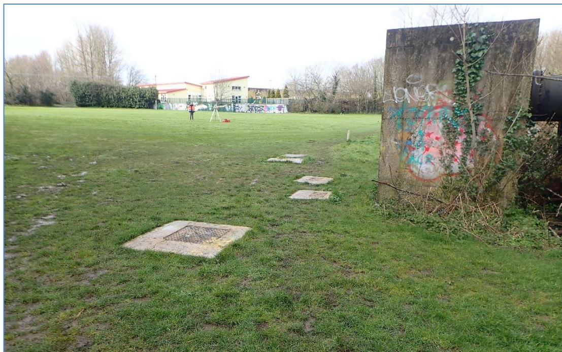
Plate 11: Service boxes to facilitate the water pipe, off the south bank.
